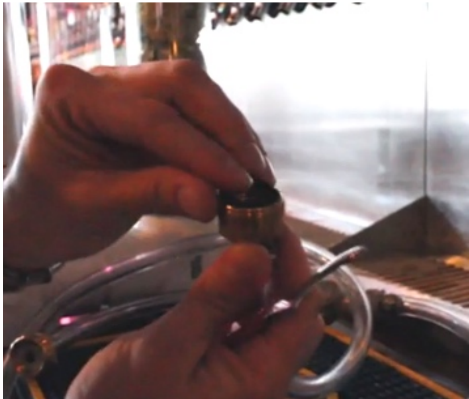
Figure 5: Inserting Washer into Hose
